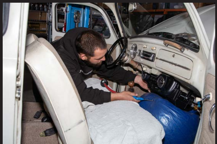
The mounting bracket for the evaporator unit are pre-drilled, and the unit itself are installed. Sean uses a partially inflated exercise ball to hold the unit in place during install.
